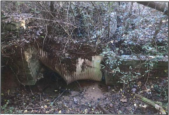
CP16 Photo 1 (66°) View of an old outfall pipe and headwall structure located at the stat of the perennial stream. (33.69398N, -84.15412 W)
