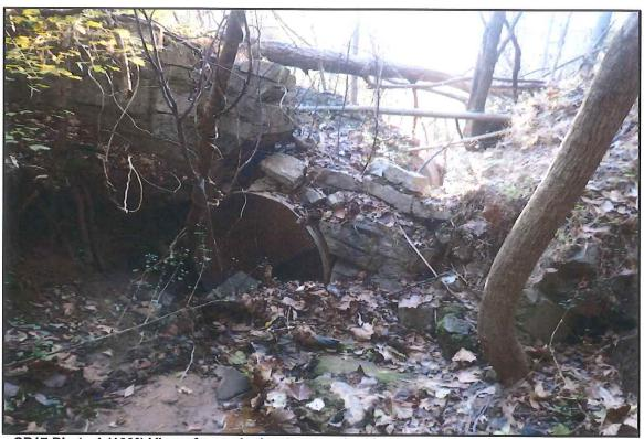
CP17 Photo 1 (109°) View of a washed out cart path culvert crossing on the perennial stream. (33.69367 N, -84.15401 W)
