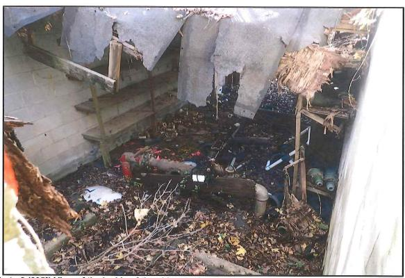
CP22 Photo 2 (235°) View of the inside of the old pump house structure. View is through the roof which is failing. (33.69184 N, -84.1513 W)
